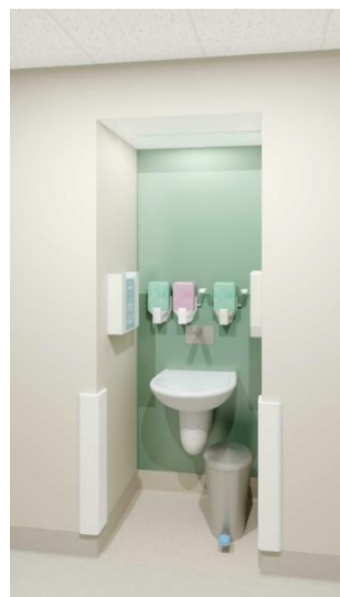
Figure 1.9: Reduced height ceiling within a corridor bay
